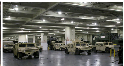
Cargo Hold Lighting
