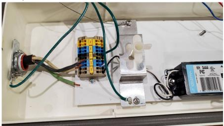
6. Make connections in terminal block by actuating the internal levers with a thin, flat blade screwdriver or similar tool.
