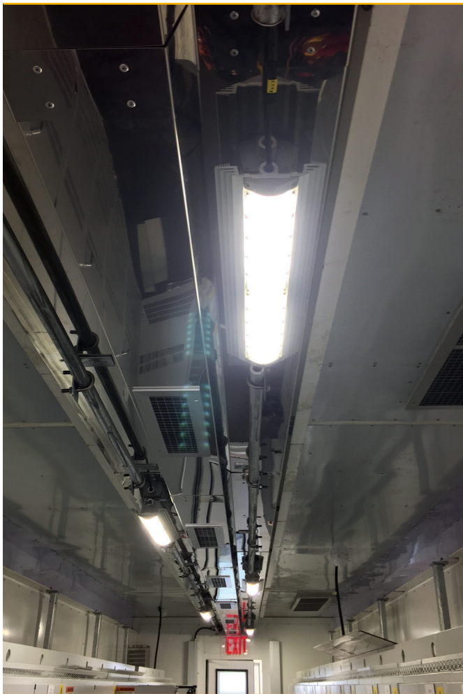
HDL2s in an electrical control room
