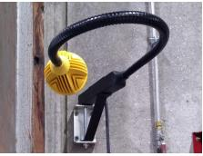
**4.** Aim the fixture and use the mounting bracket to swing the fixture in and out of the way as necessary.
