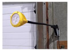
1. Position the fixture with the arm in a straight line.
