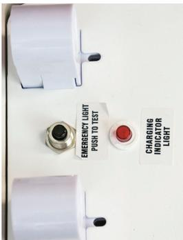
When AC power is applied, the charging indicator light will illuminate, indicating that the battery is being charged.
