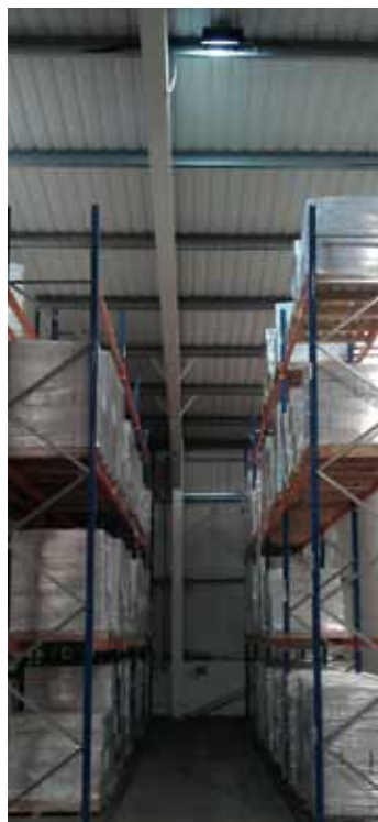
Illumination difference: on the left, an aisle lit by a 400W HPS lamp; on the right lit by a GlowLED 160W LED lamp
