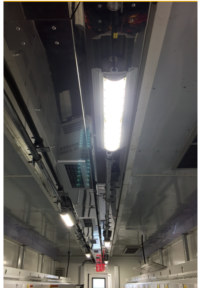
HDL2s in an electrical control room
