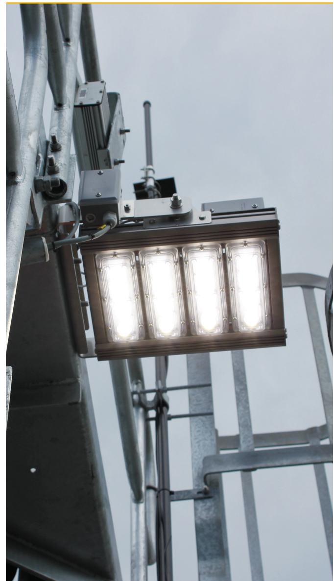
EcoMod 150 on an RTG crane
