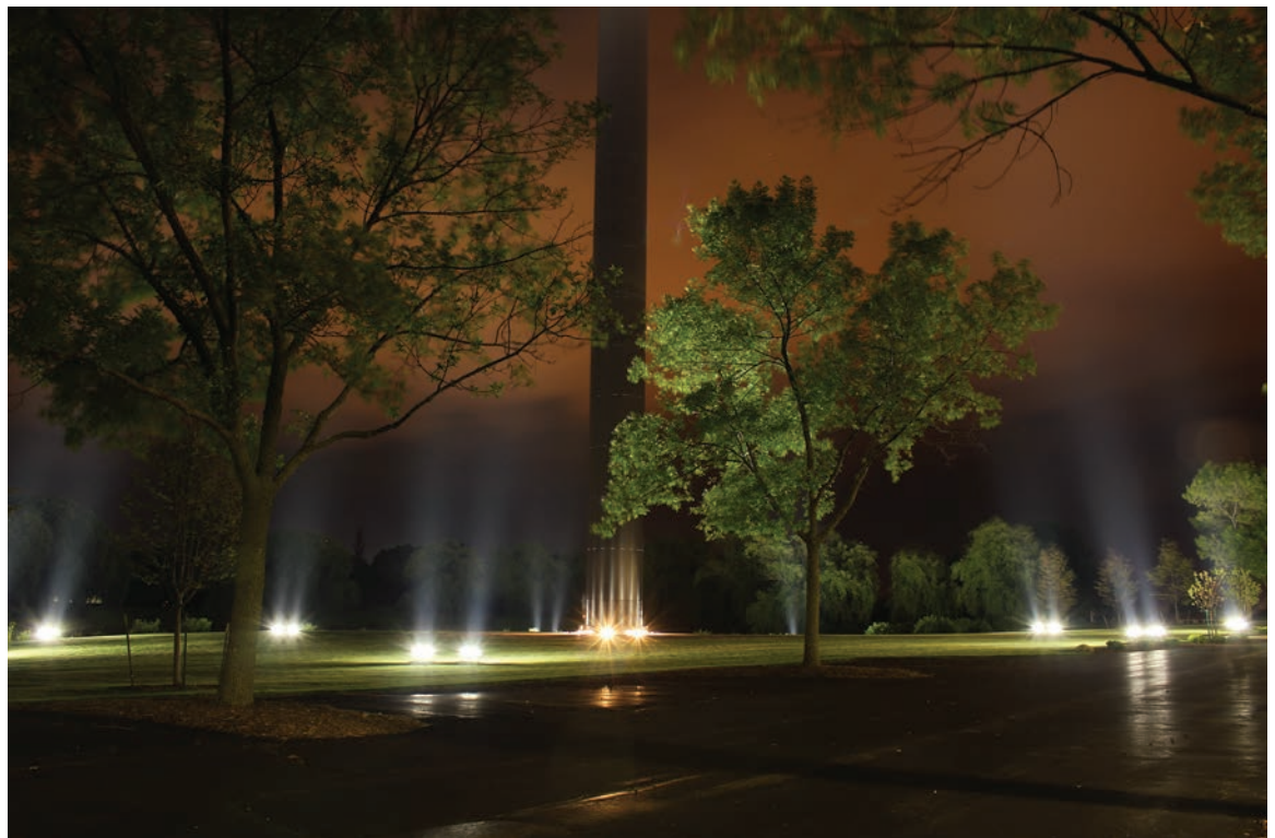
In a radius of 55 ft. from the flagpole, fixtures are aimed 22 1/2 deg. to either side of the pole and about 6 deg. down from vertical. This lights the entire flag regardless of wind strength and direction.
