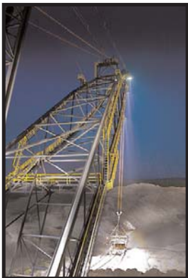
A specially-colored lamp emphasizes the color of the matrix, helping operators discern ore from overburden.
